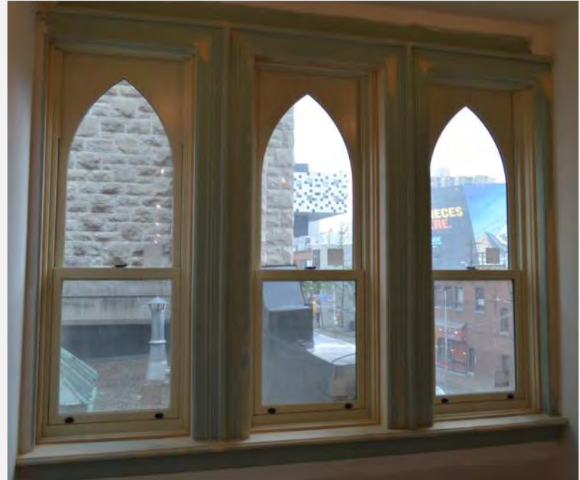
Step 6: New windows go into existing refurbished historical trim
