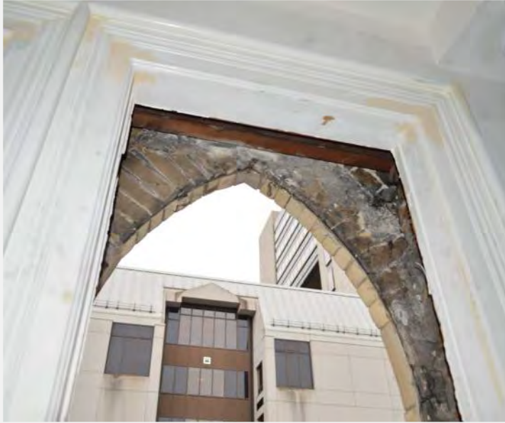
Step 3: Opening is exposed from interior
