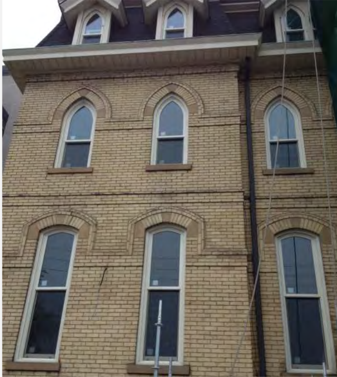
Step 5: New windows are anchored, foamed and blocked
