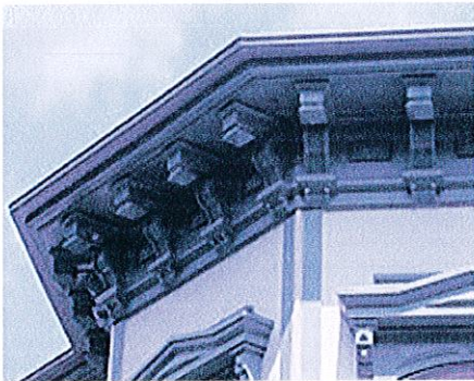
Photo of similar detail required to restore brackets.
