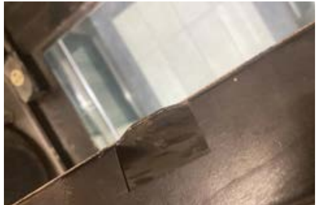
Ceiling hatch pushed hard enough to bend the metal that keeps the door closed.
